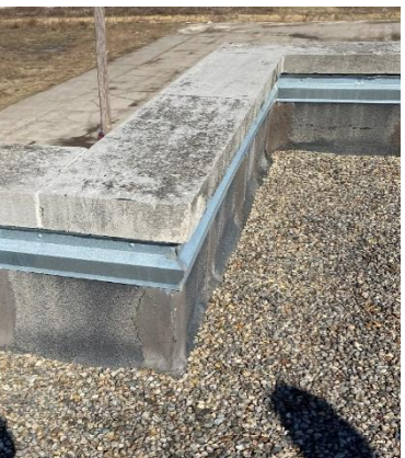
parapet, coping, and flashing
