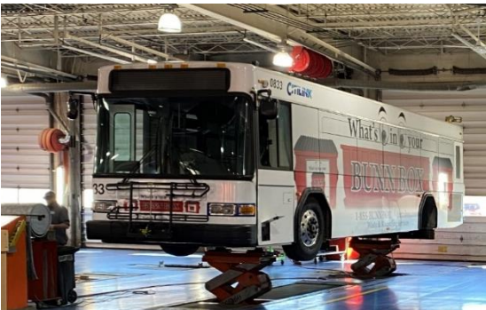
Figure D-46: In-floor lifts
