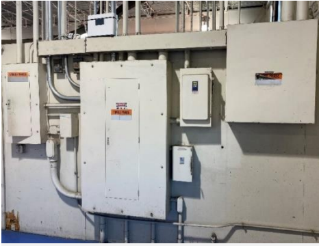
Figure D-60: Service entrance and distribution
