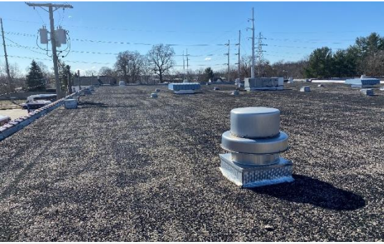
Figure D-43: Storage barn roof
