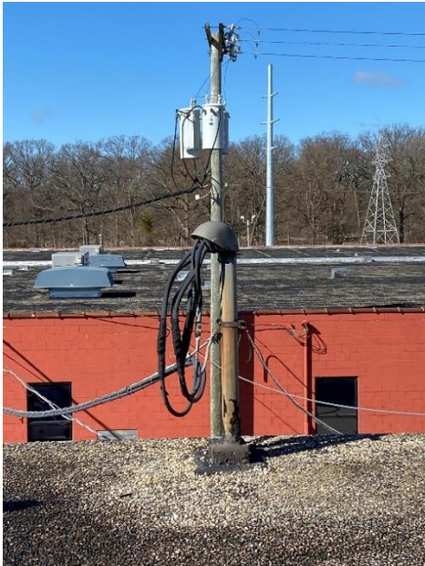
Figure D-61: Utility pole, transformer, and weather head
