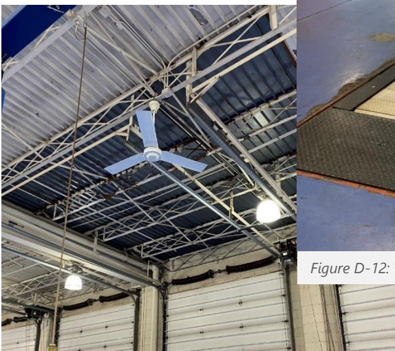
Figure D-11: Area of roof deck replacement.
