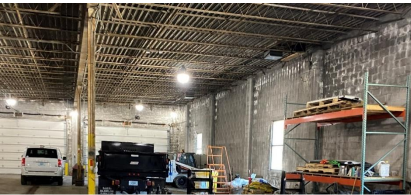
Figure D-45: Storage barn interior
