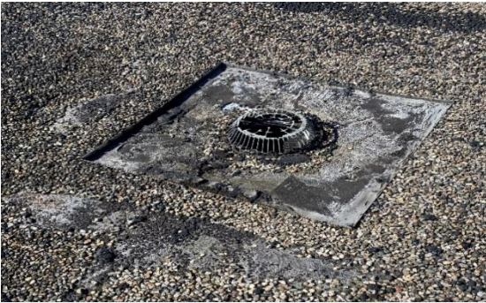
Figure D-44: Storage barn roof drain
